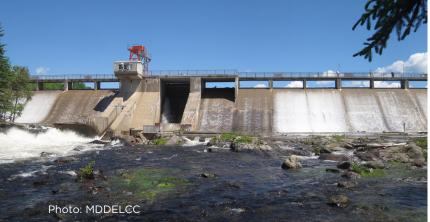
This summer, Brookfield will be completing the refurbishment project at the Kiamika dam that was built in 1952 and is about 40 km northeast of Mont-Laurier. The two three-metre square sluice gates, which are used to allow water flow on either side of the dam, have been refurbished, along with the equipment that operates them.
